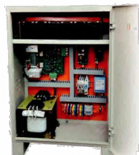
Automatic Rescue Device (ARD)
